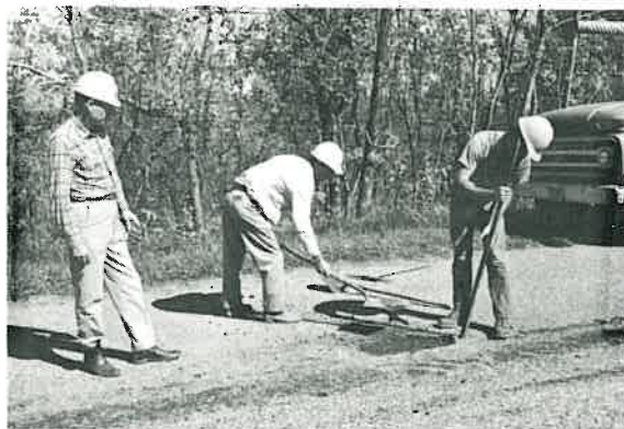
Harrison Heath, area foreman of Polk County, looks on while James Golden and Dennie Rowe shovel out material to make tests in an area where a water problem has hindered construction on Skyline Drive (Highway 88).
